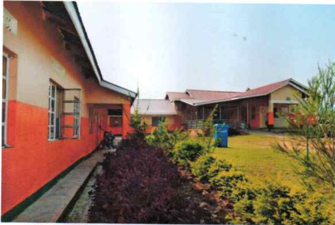
Transformation of infrastructure. The building on the right hosts the scan room
